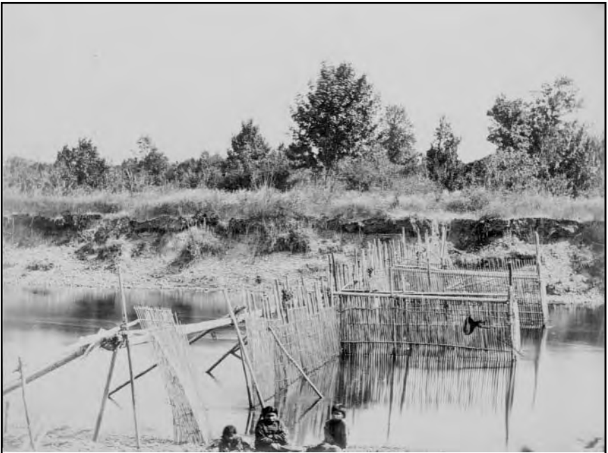
Salmon weirs on the Cowichan River, Vancouver Island, BC, circa 1870. Photograph by Frederick Dally. Library and Archives Canada, negative C-010334
